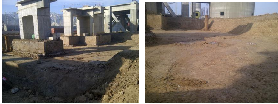
Figure 6. The area of unloading of the soil mass from the embankment
