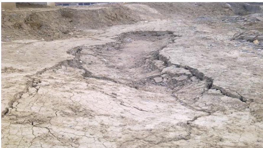
Figure 1. Self-compacting of bulk soil at a construction site
